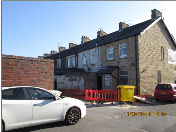
Application site, rear of property
